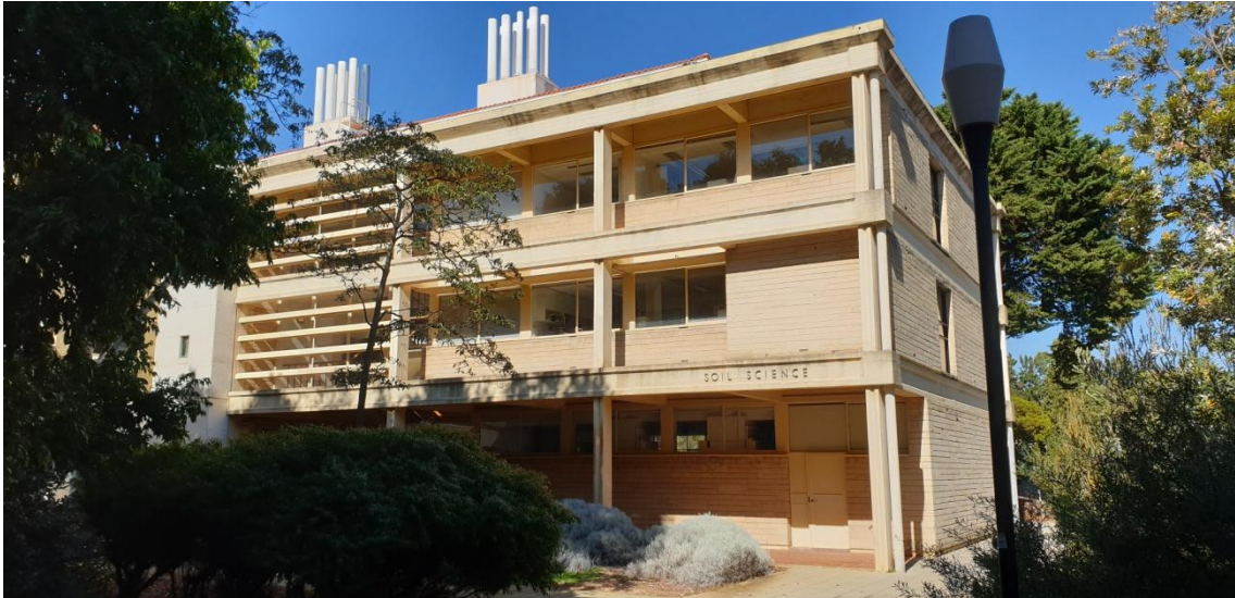
Soil Science Building of 1968 at University of Western Australia, Crawley. (John Taylor 2019)
