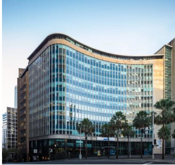
Qantas House, designed by Rudder Littlemore & Rudder and built in 1950 at 1 Chifley Square Sydney (Darren Bradley photo, Docomomo Australia)
