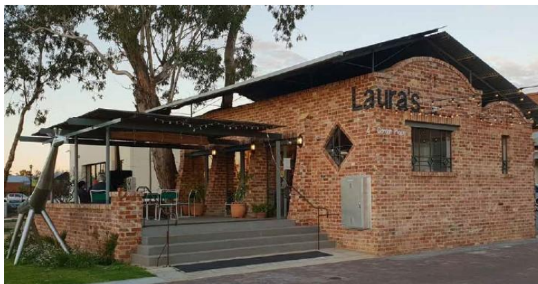
Wine Bar at Northam ( The Architect , Spring 2019, p.36).
