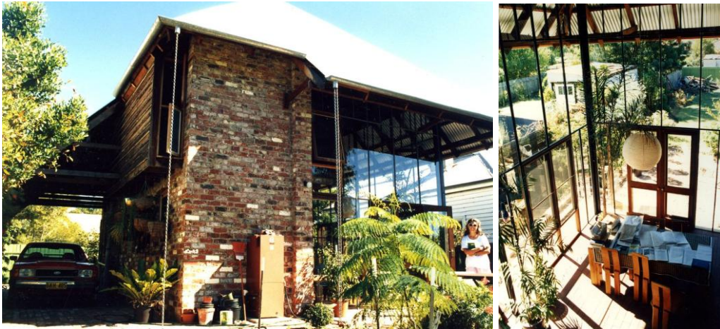
1983 Hopetoun Terrace House ( Architecture Australia , September 2012).
