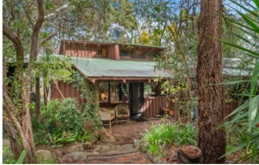
1975 – 15 Michael Crescent Boya (2025, realestate.com.au)
