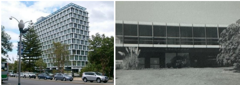
1963 Council House Perth (Wikipedia); 1964 Waller Residence at 282 West Coast Highway Scarborough shown in 1971 (Julie & Sam Ruiz)
