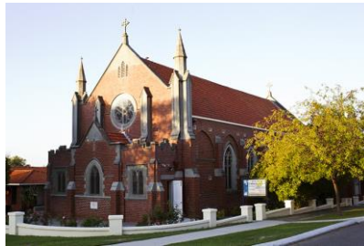
Holy Rosary Church, Thomas Street Nedlands built in 1936 ( http://www.holyrosarynedlands.org.au/Buildings.html )
