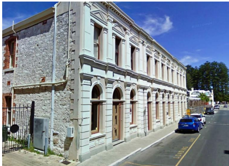
Lilly's Buildings 34-42 Cliff Street Fremantle of 1896 (Google 2013)
