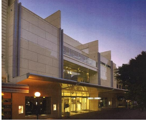
Hay Street façade of David Jones store at Perth (Kym MacCormac)
