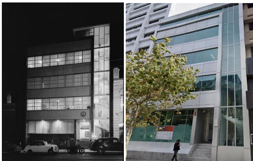
South British Insurance Building 23 Barrack Street Perth (1958 SLWA 239839PD; 2024 Google)
