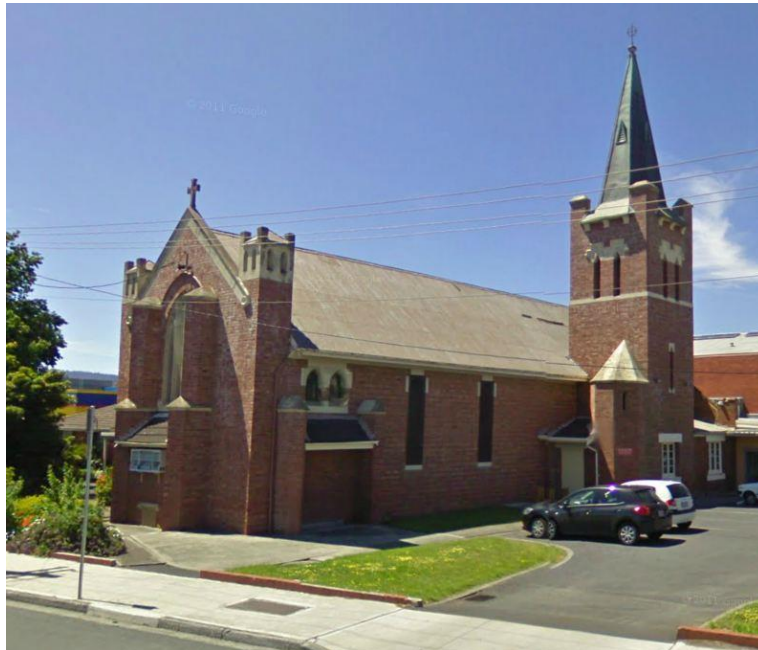
St Mary's Church, Springfield Avenue, Moonah, Tasmania of 1924 (Google 2012)
