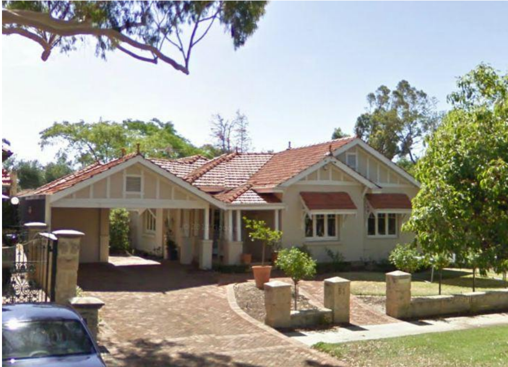
Stein designed the residence at 51 Thomas Street, Nedlands built in 1925 for widow Mrs Elizabeth F. Telford. The carport at left is a portion of 1994 alteration and addition works by John Taylor (Google 2013)
