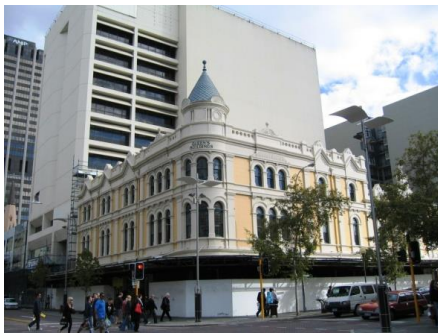
3 rd floor etc, Queen's Buildings, cnr William & Murray Sts Perth (John Taylor 2008)
