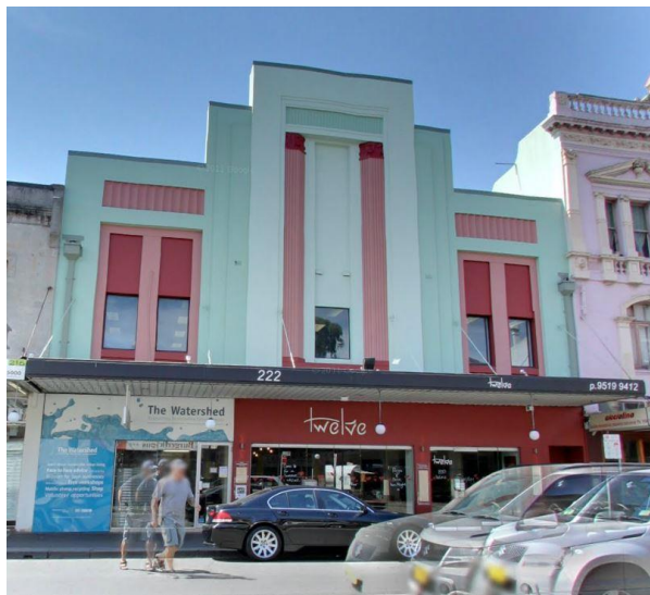
Former Hoyts Theatre in Newtown, Sydney of 1934 (Google 2013).
